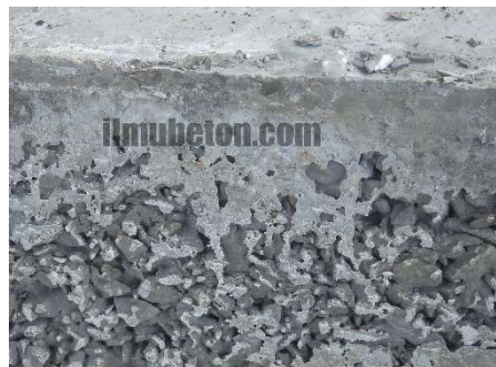
Gambar 2.20 Proses Segregation
