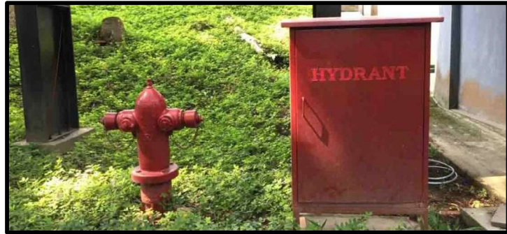
Gambar 5.11 Fire Hydrant
